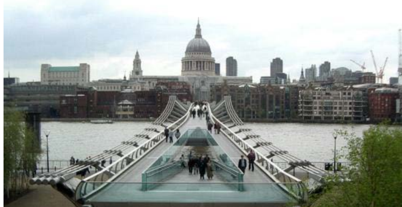
Figure (6) London Millennium Bridge
