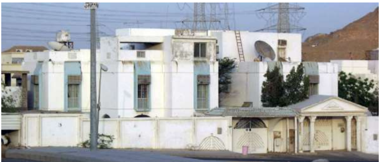
Figure (4) A typical dwelling of the project
